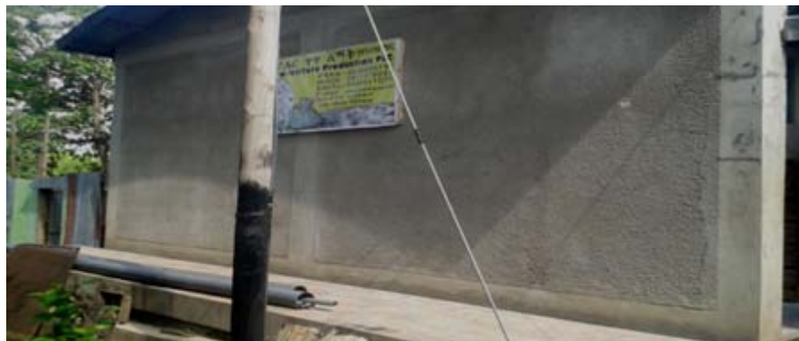
(c) Concrete (asphalt) floor and corrugated iron roof house
