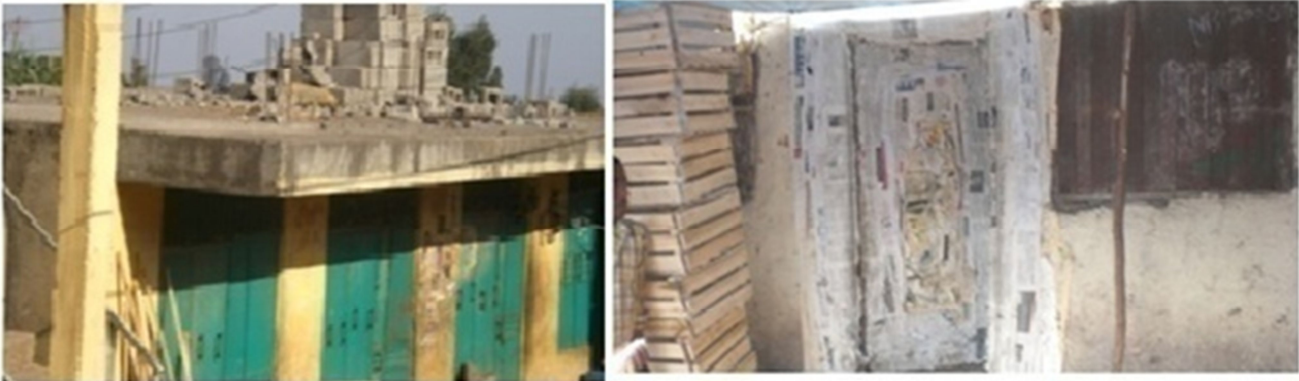
Annex Figure 9.2.12. Banana ripening chambers at regional/central wholesale markets air-tightly sealed (for 2-3 days) after loading and kerosene smoking for ripening initiation
