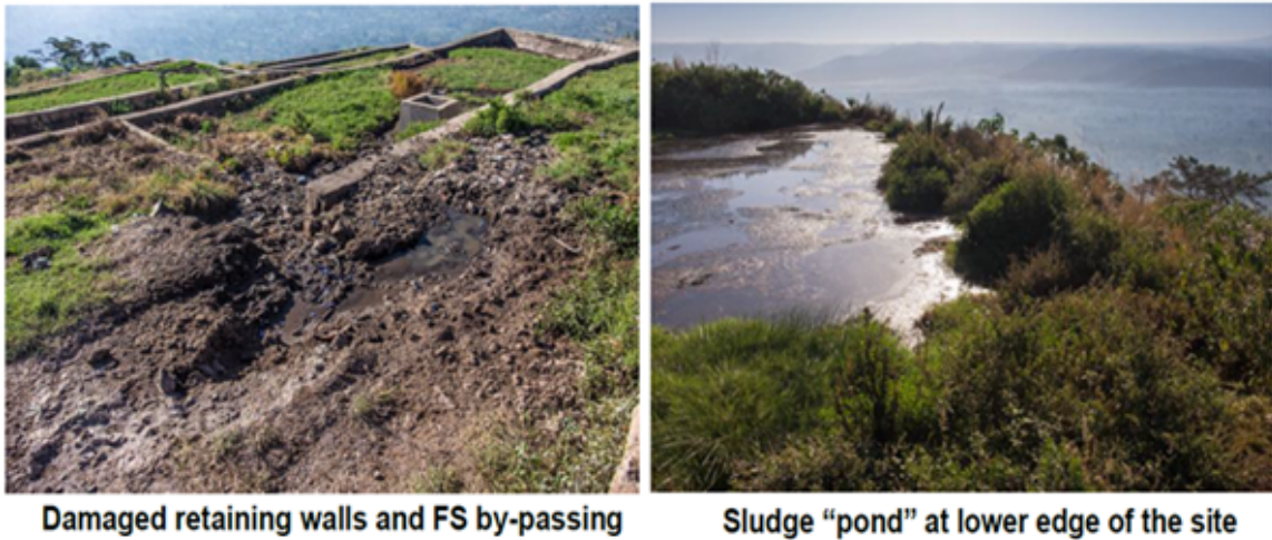
Figure 5: Conditions of FS drying beds in rainy season in Hawassa Ethiopia
