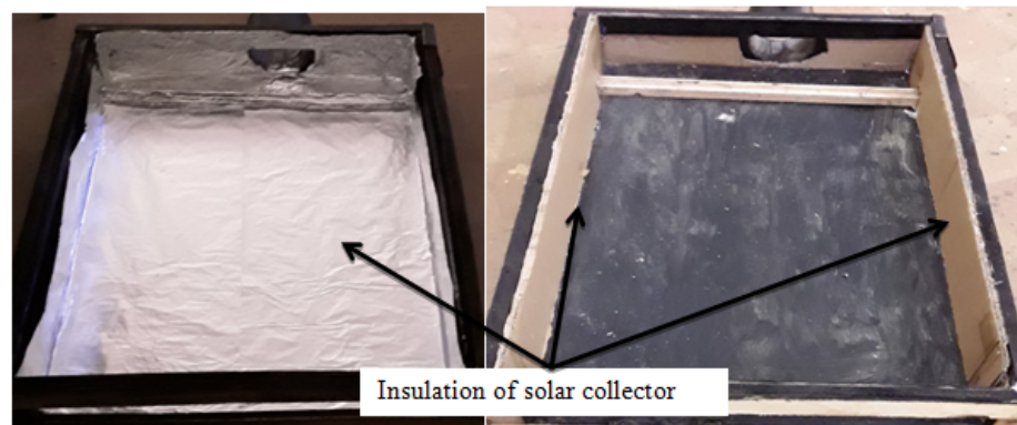
Figure 15: Insulation of non-transparent parts of solar collector
