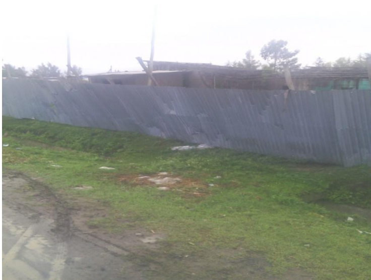
Figure 4.16: Constructions under Demolishing (Photo by the Researcher, April, 2016)
