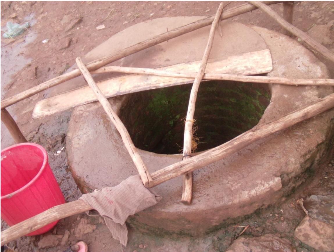
Figure 3. Unprotected well found in Ginjo guduru kebele near Jimma University
