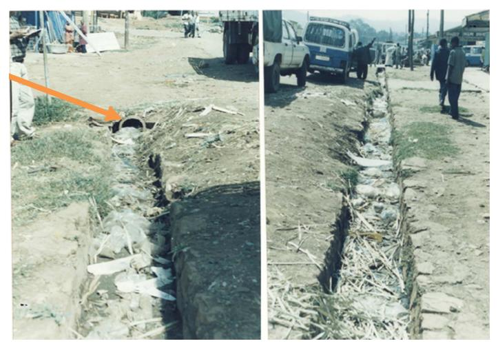
Figure 3. Plastic bag wastes clogging sewerage lines (or drains) (in Jimma City).
