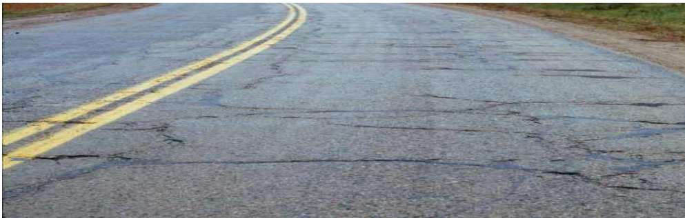
Figure 2.9: Block Cracking
