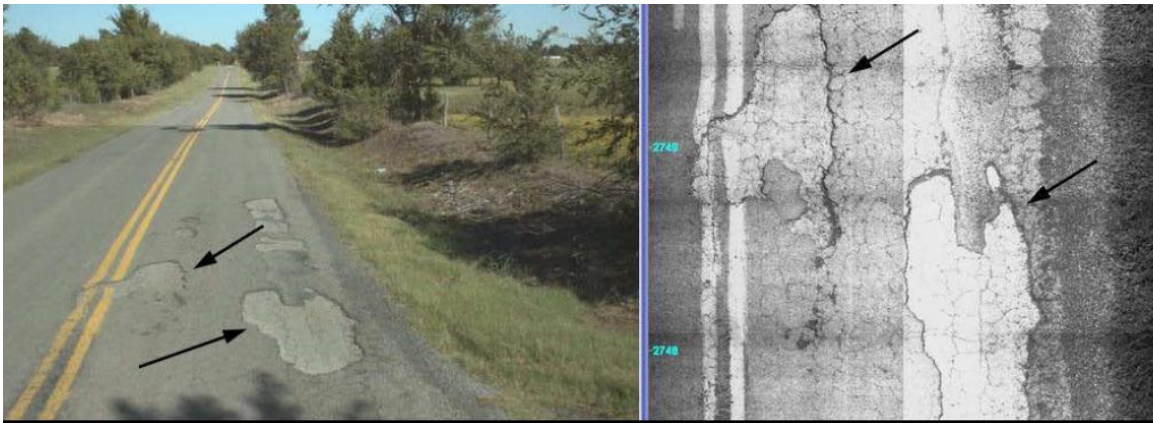
Figure 2.5: Delamination
