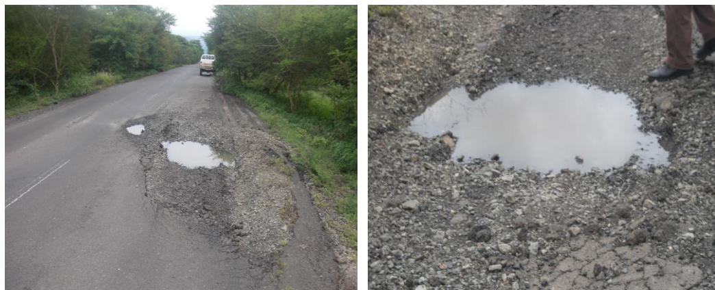
Figure 4.28: Base Failure
