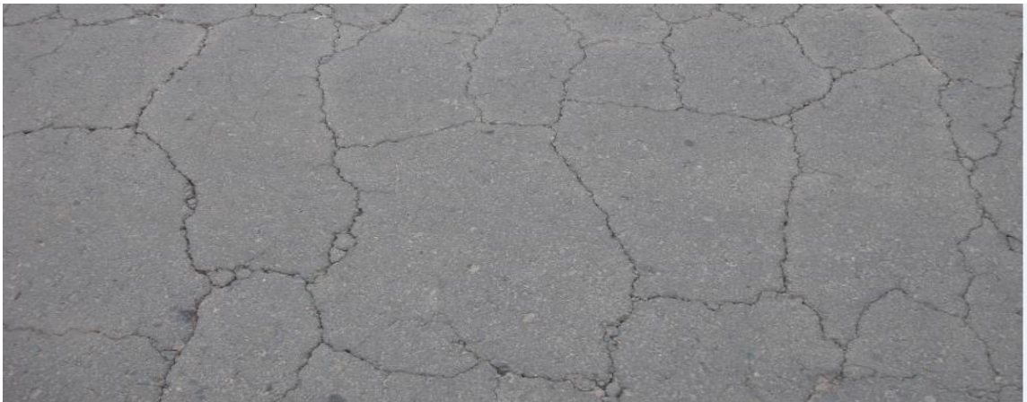
Figure 4.17: Block Crack
