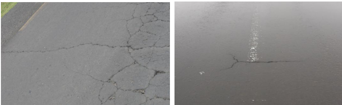
Figure 4.19: Transverse Crack
