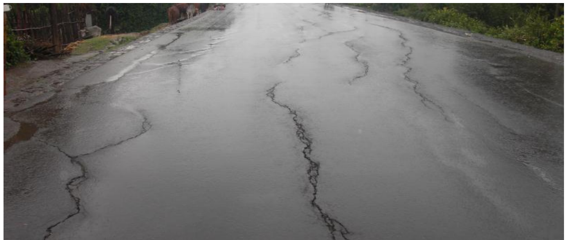
Figure 4.18: Longitudinal Crack
