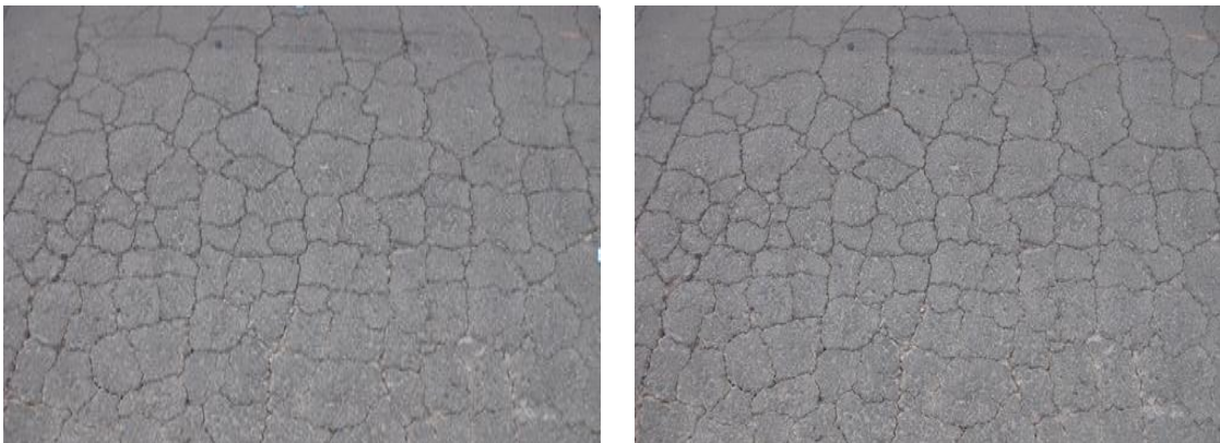
Figure 4.16: Alligator crack
