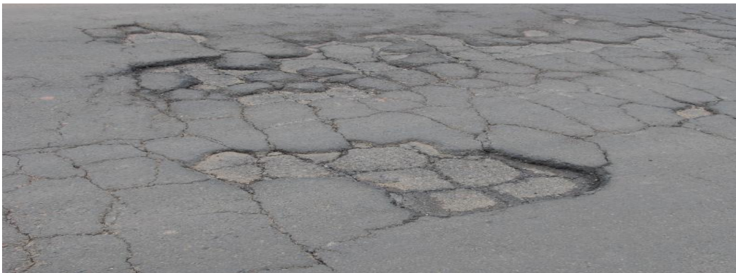
A. Patching on existing crack
