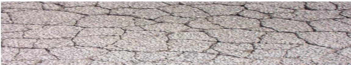
Figure 2.3: Alligator Cracking
