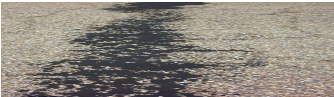
Figure 2.6: Bleeding or Flushing
