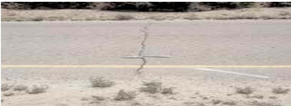
Figure 2.2: Transverse Cracking
