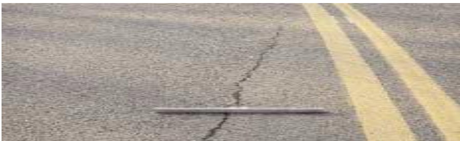
Figure 2.1: Longitudinal Cracking
