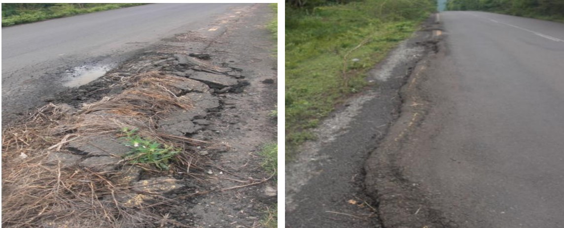
Figure 4.23: Edge Damage
