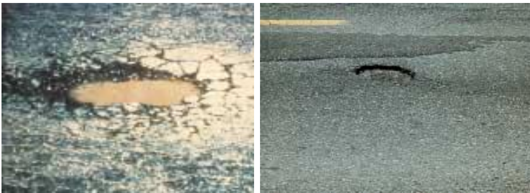
Figure 2.4: Potholes
