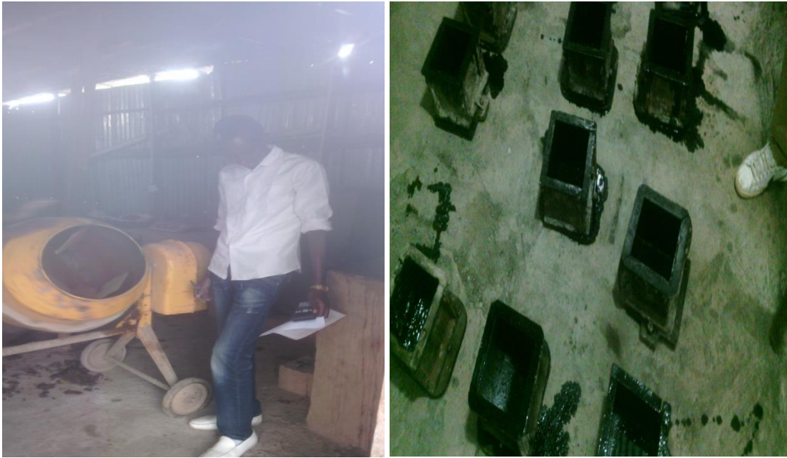
12. During mixing and preparing cubes
