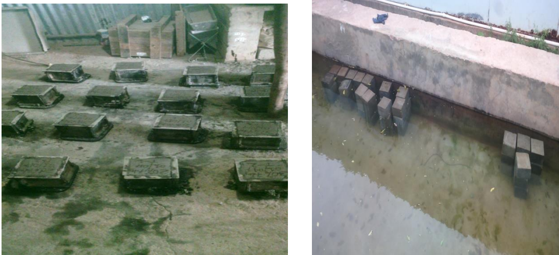
13. Casting and curing
