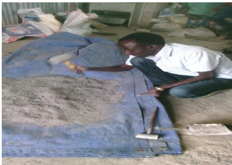
Fig.1.2. Manual grinding of calcined termite hill clay
