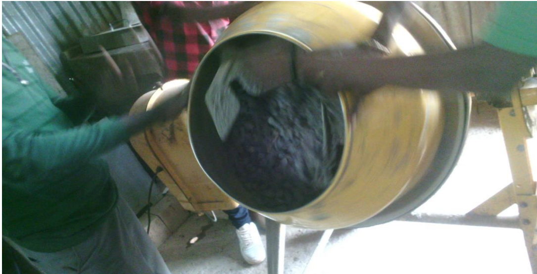
Fig 3.2. Dry mixing of concrete ingredients
