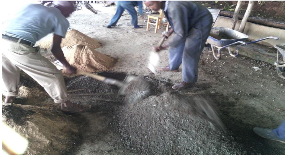
Figure 3.3.7 dry mixing of material
