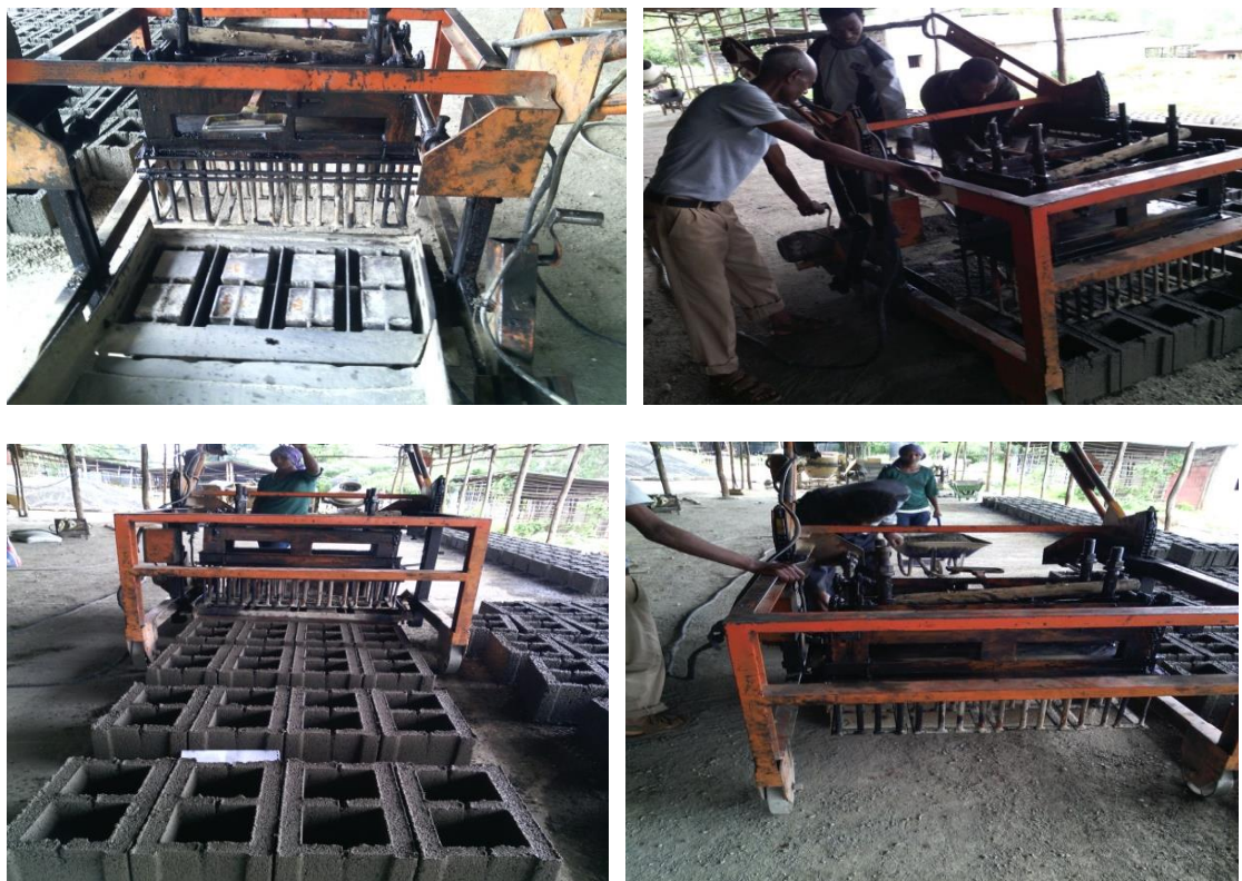
Figure 3.3.8 casting of HCB
