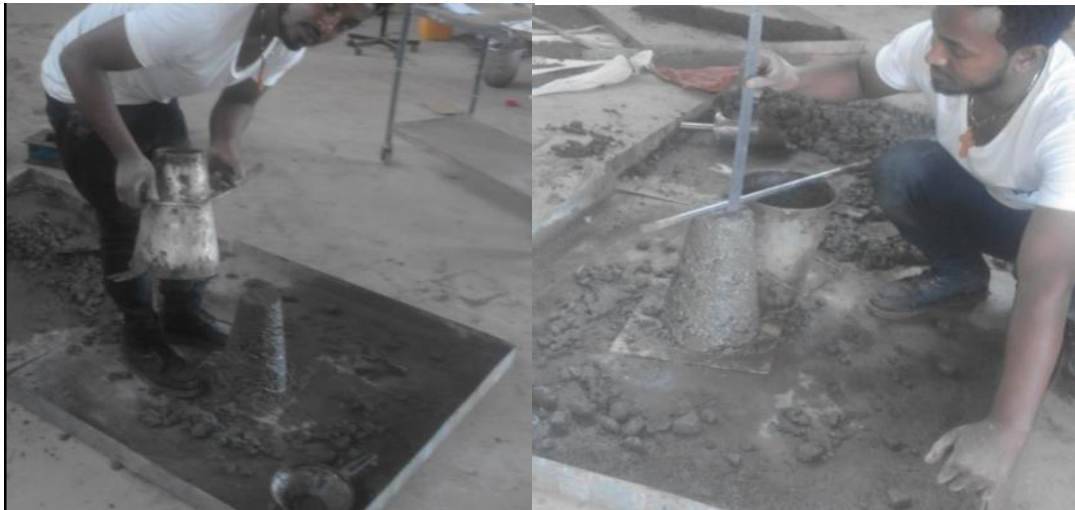
Figure 3.3;A and B shown the slump cone test of concrete workability
