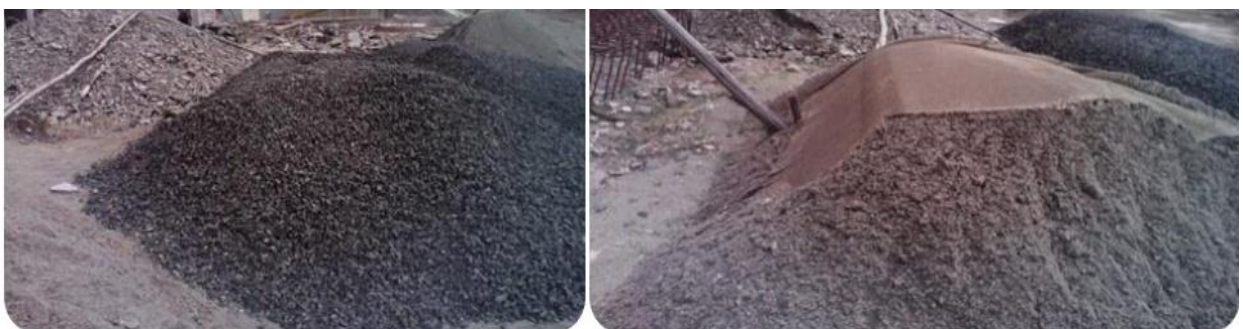
Figure 4.13 Proper handling of sand and coarse aggregate on building site
