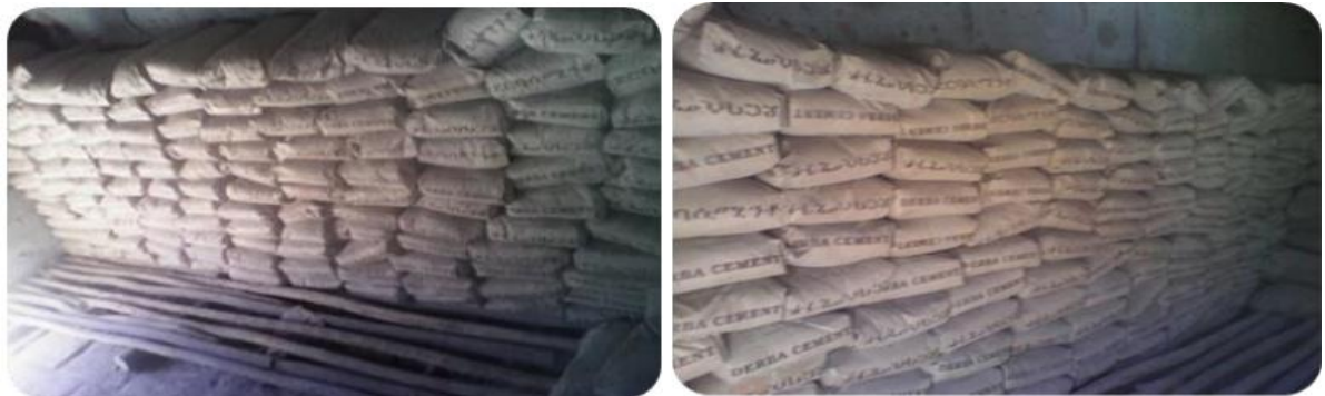
Figure 4.11 Recommended ways of storing cement on building site
