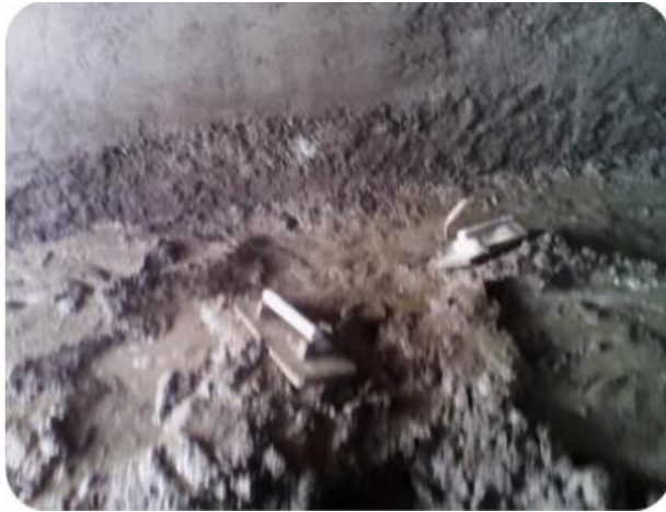
(a) Excess cement mortar left on site
