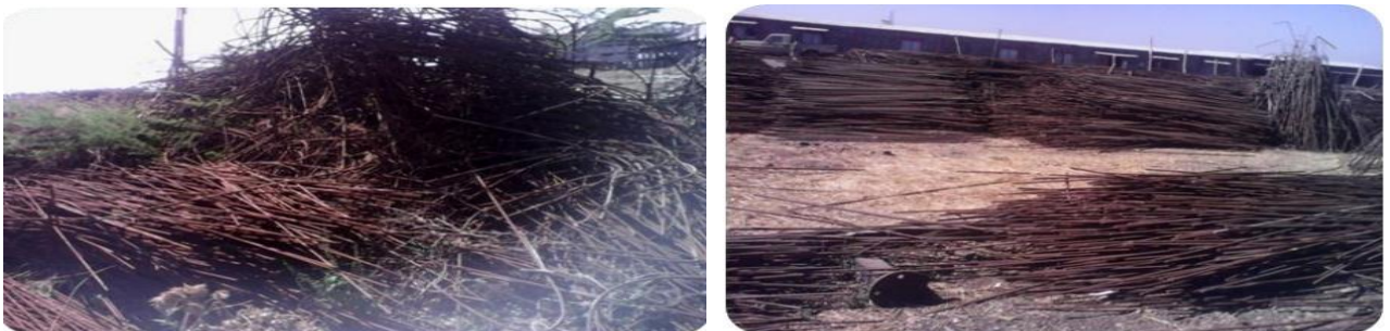
Figure 4.14 Wastage of steel reinforcement bar due to Non-optimized cutting of bars and design change
