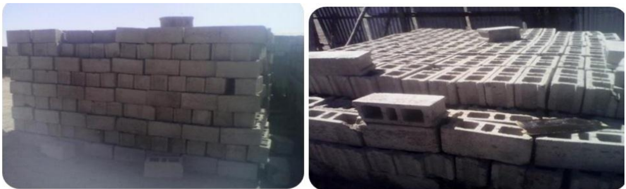
Figure 4.12 properly packed HCB on building construction site
