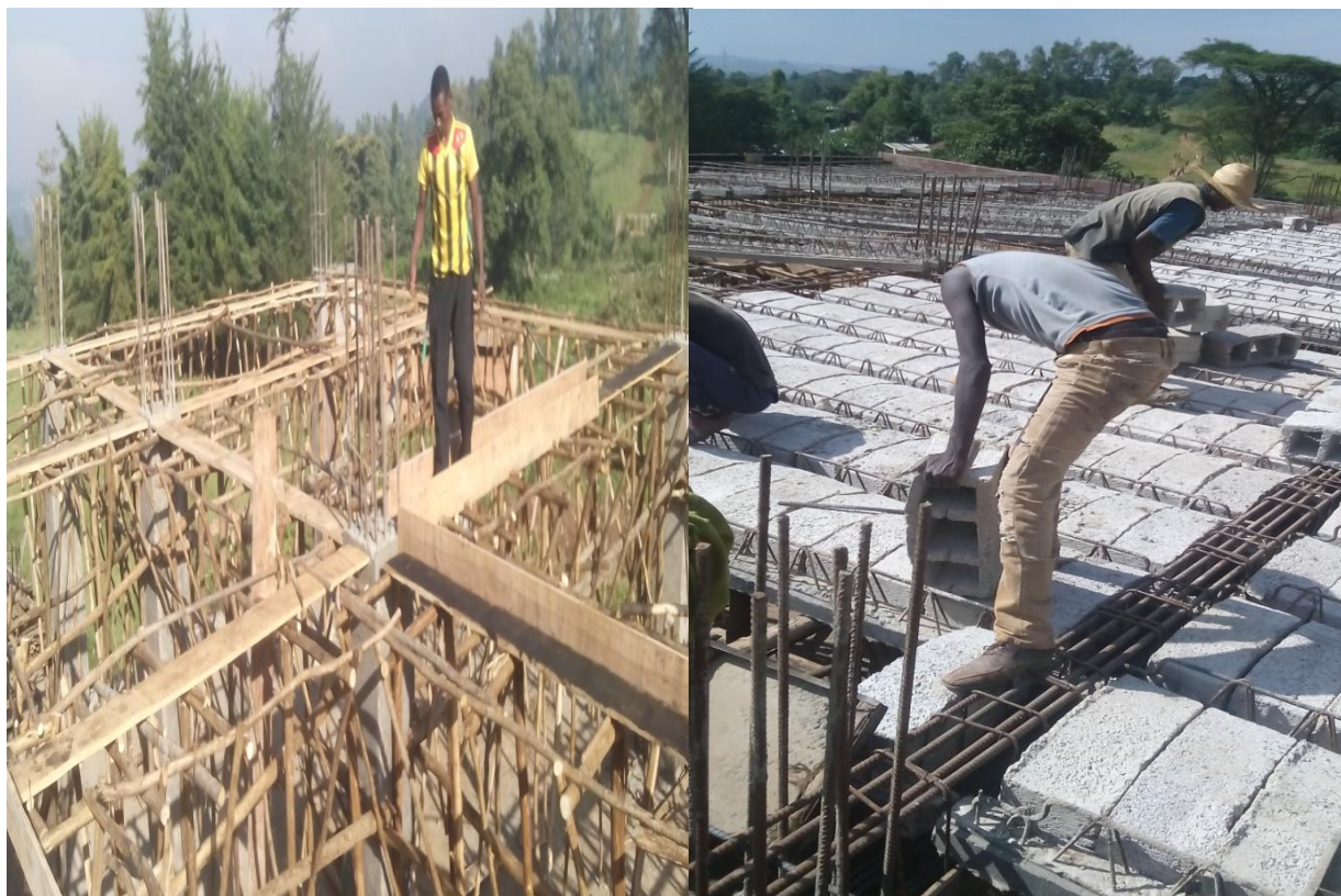
Figure 2.1:Formwork for ribbed slabFigure 2.2:Ribbed slab under construction
