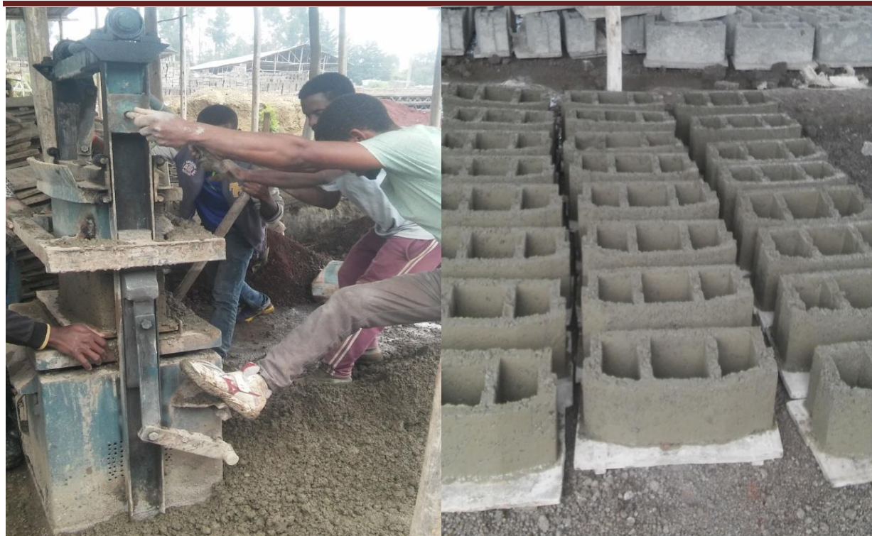
Figure3: 9 Compacted and placing Ribbed HCB
