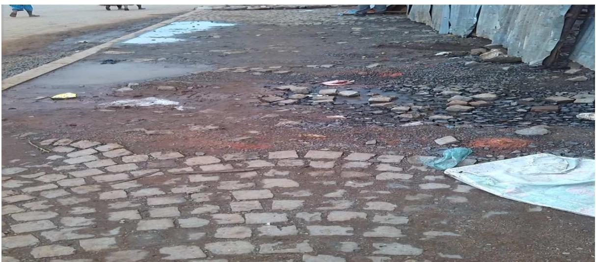
Figure 1.3: Jimma Town cobblestone pedestrian sidewalk constructed on 2006
