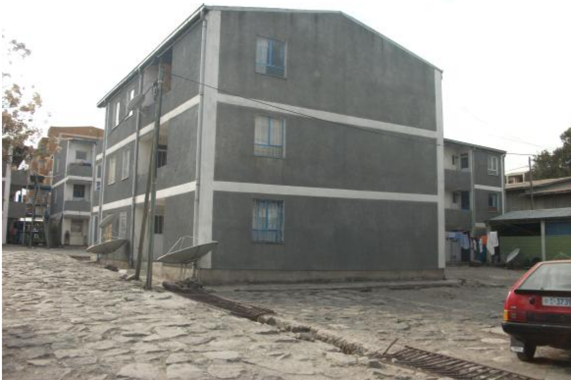
Photo 3: Signal Site Condominium Houses
