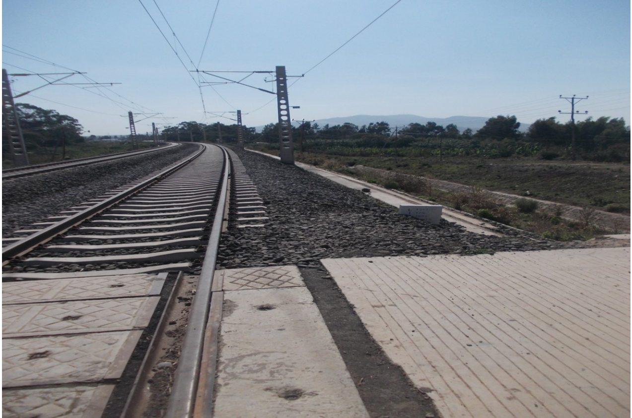
Figure 4.25 Railway Field survey, April 2017
