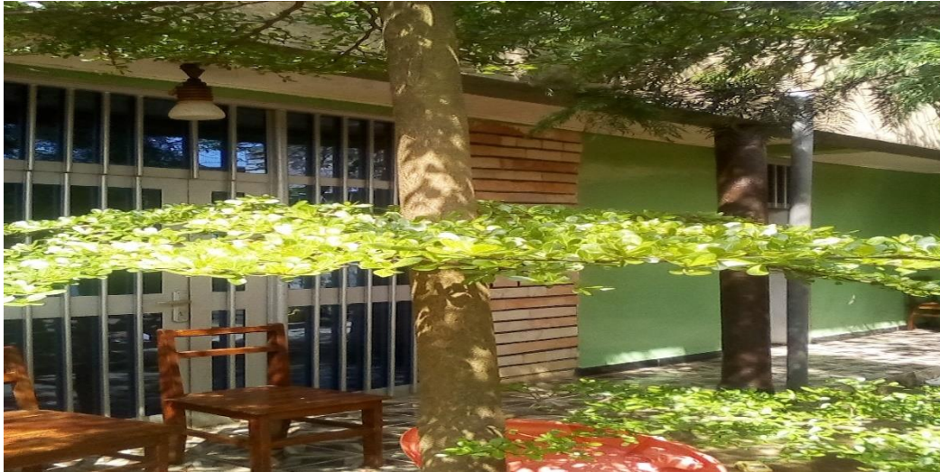
Figure 4 The good structure of the wall of the house
