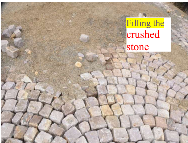
Figure 9 The different stages of cobbleston pavement
