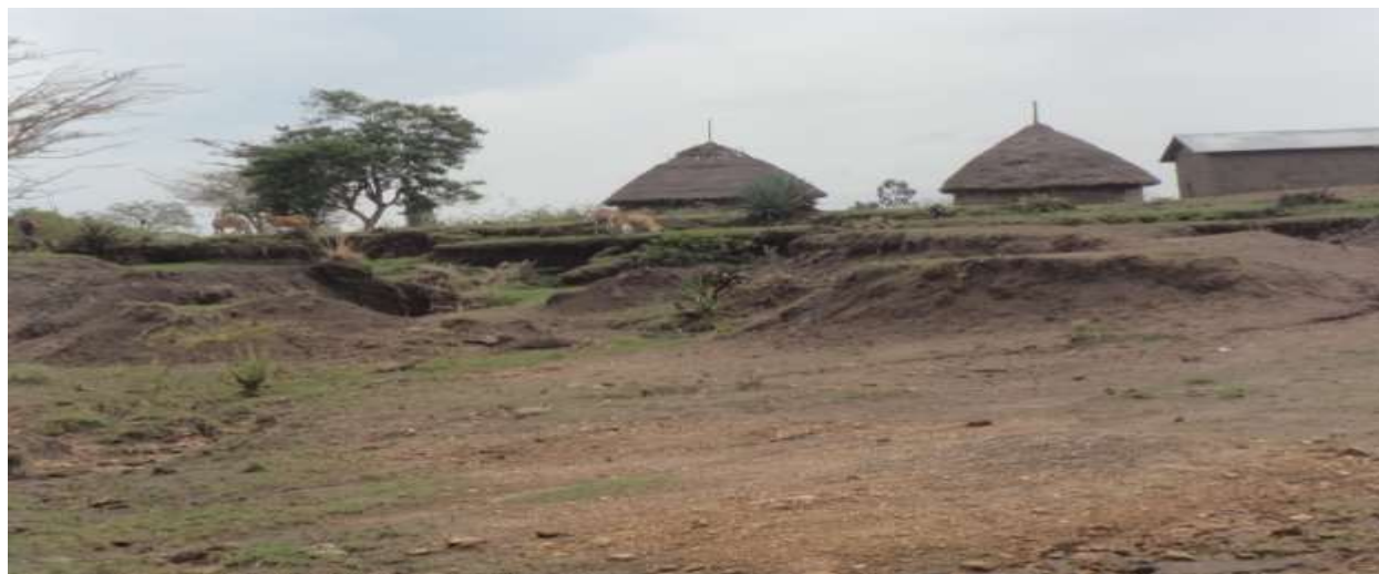
Figure 14: Degraded land in bonsha keble in shashogo woreda (photo by Author)
