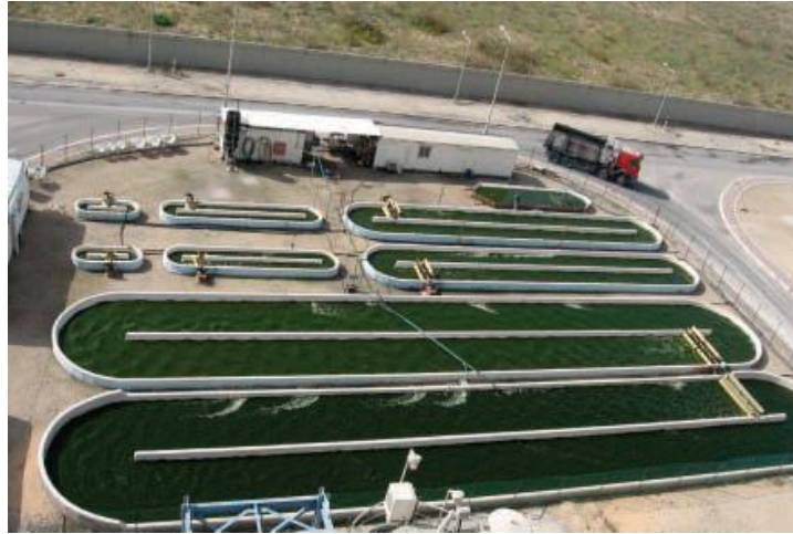
Figure 2.5: The pond microalgae production plant (adapted from: Demirbas, 2008).
