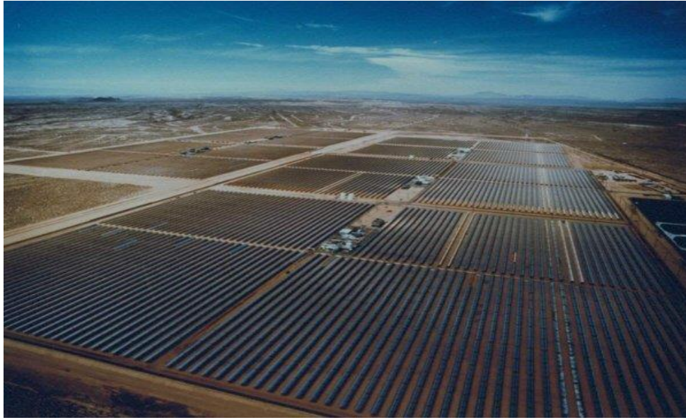
Figure 1.1 Aerial view of SEGS III, IV, and V, three of the Luz plants located on the Mojave Desert of southern California. Photo courtesy of Luz International, Inc [3].
