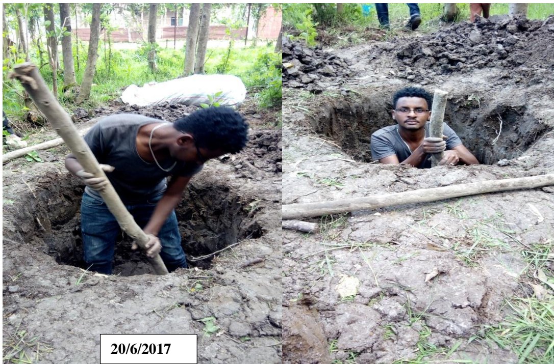
Figure 3.3: An overview of test pits (photo captured by sadiq A).
