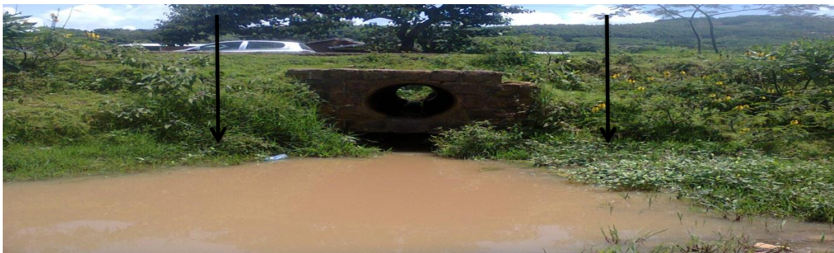
Figure 3.3 initially constructed one Rows of Pipe Culvert at Station 24+200
