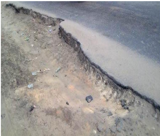
Figure 2.2a edge failure
