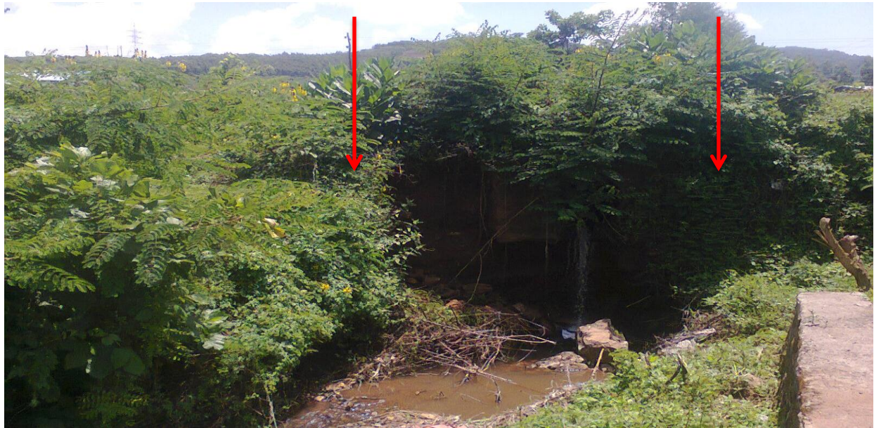
Figure 3.4 initially constructed one Rows of Pipe Culvert at Station 42+120
