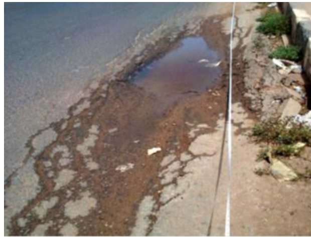
Figure 2.2 b pothole road side
