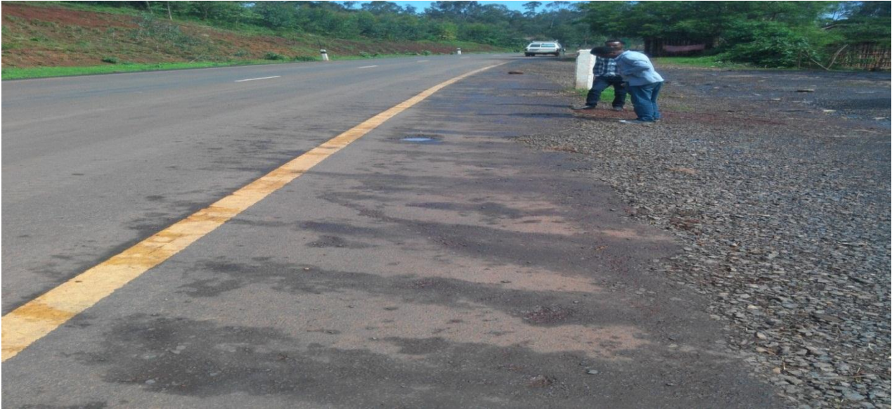
Raveling type of deterioration
