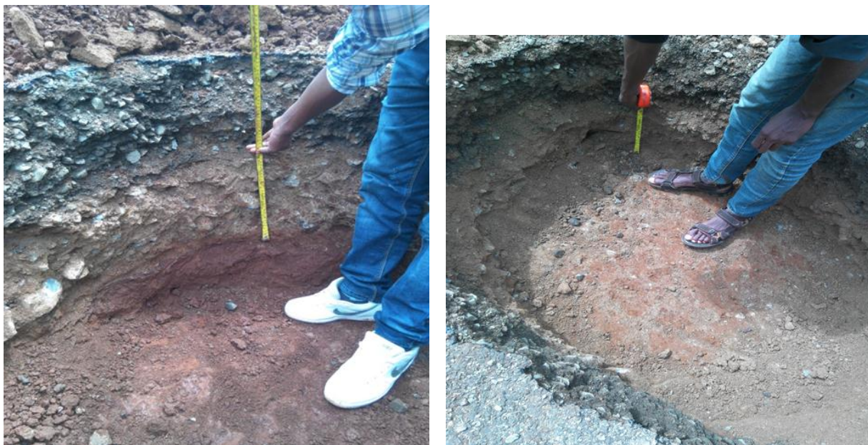
Figure 4.6 Measuring the thickness of the pavement layers (photo 22, 6, 2016-17, 8, 2016)
