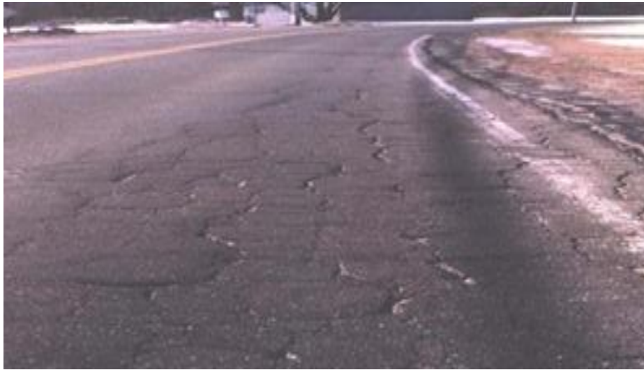
Figure 2.1 alligator crack
