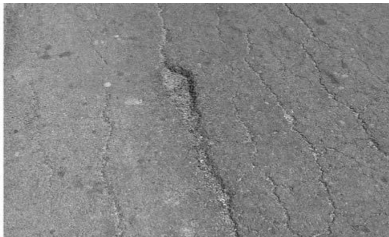
Figure 2.2 Longitudinal Cracking
