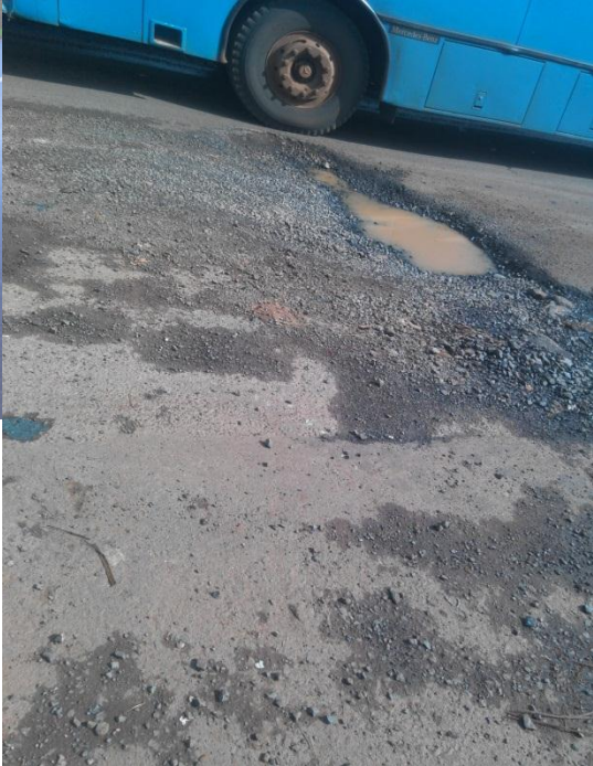
Potholes type of deterioration
