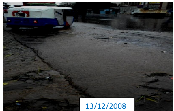
Figure-18 Cause of erosion
