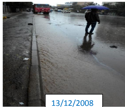
Figure-13 Road Side drain
