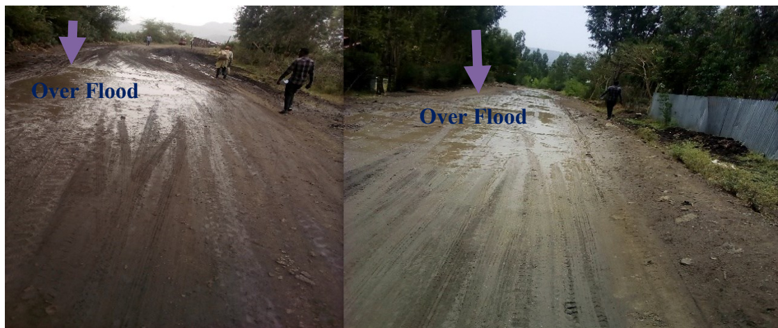
Figure 4. 21 Over flooding of water on the road by poor road drainage cross section
