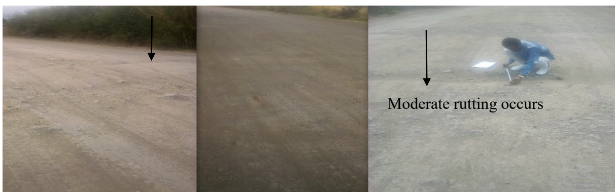
Figure 4.15 Photographs of gravel surfaced roadway in fair condition
