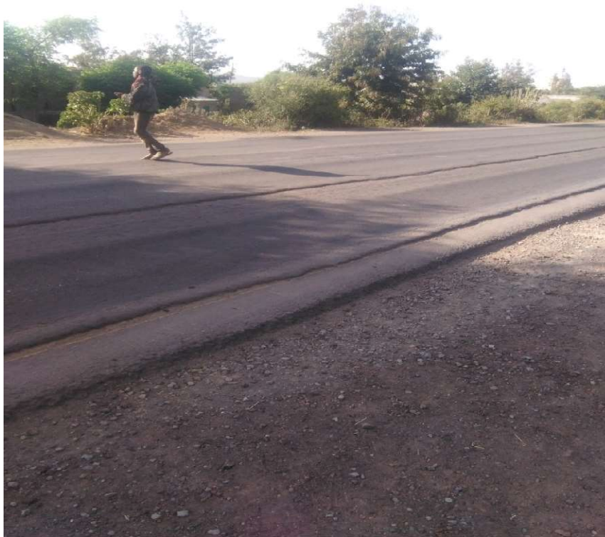
Figure4. 8 Photo shows the surface of the road segment.
