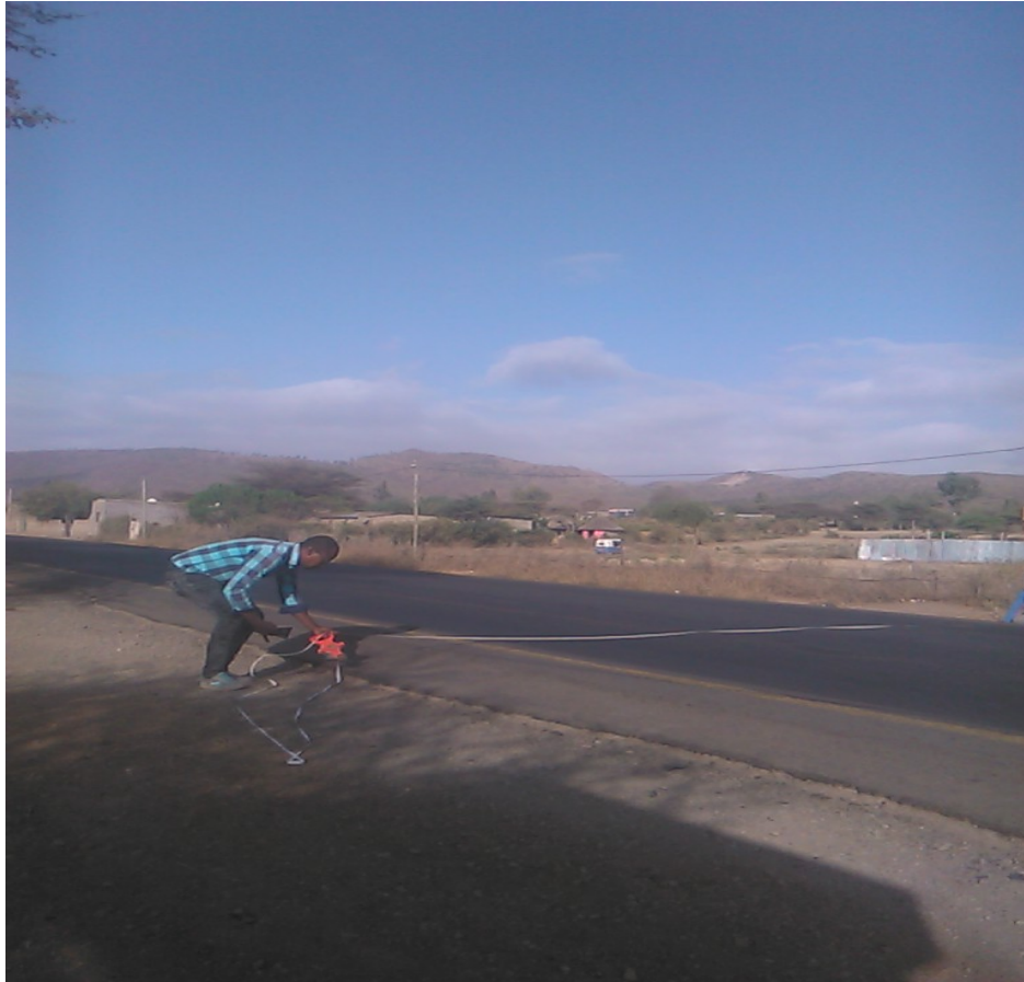
Photo shows measuring of the road segment elements.
