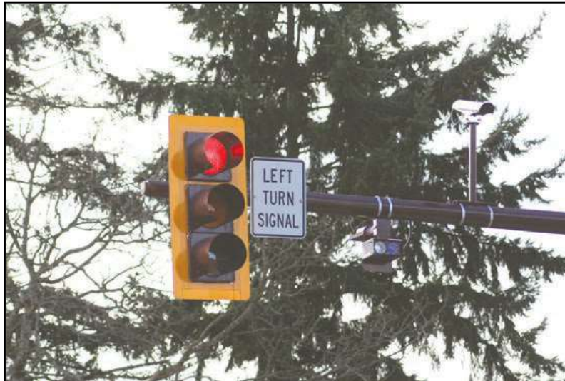
Figure 2.5: Protected Left-Turn Phasing [23]
