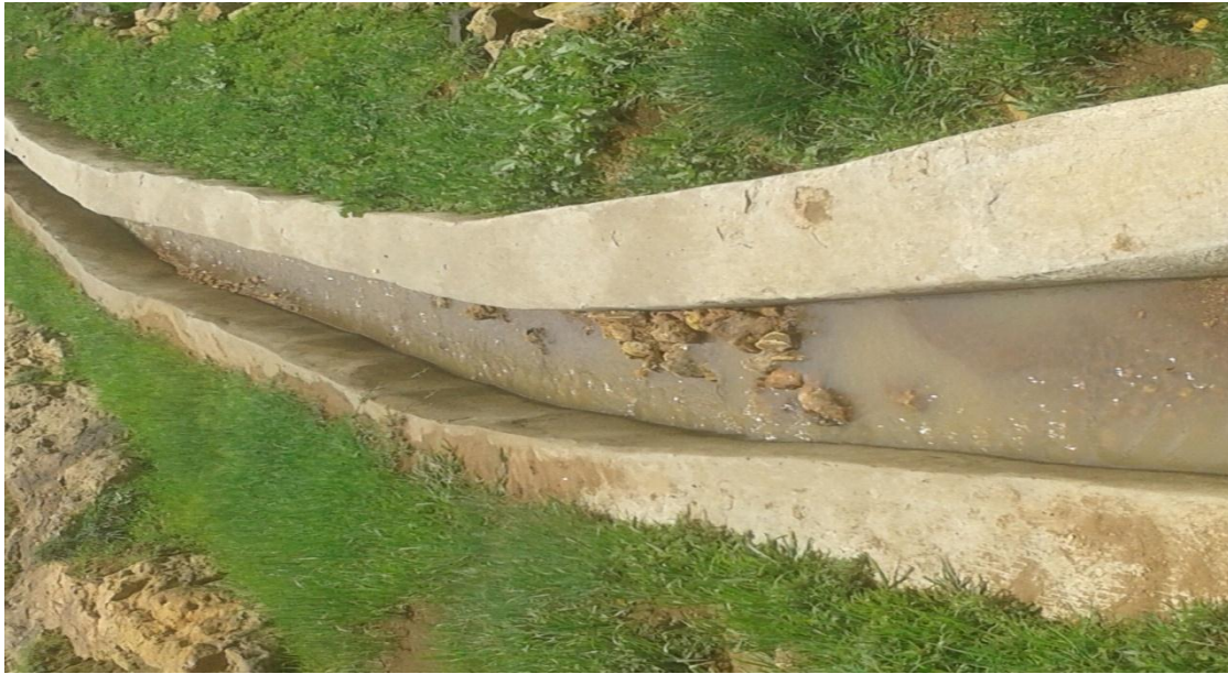
Figure: 4.7 Sedimentation problem at the canal (tankua)
