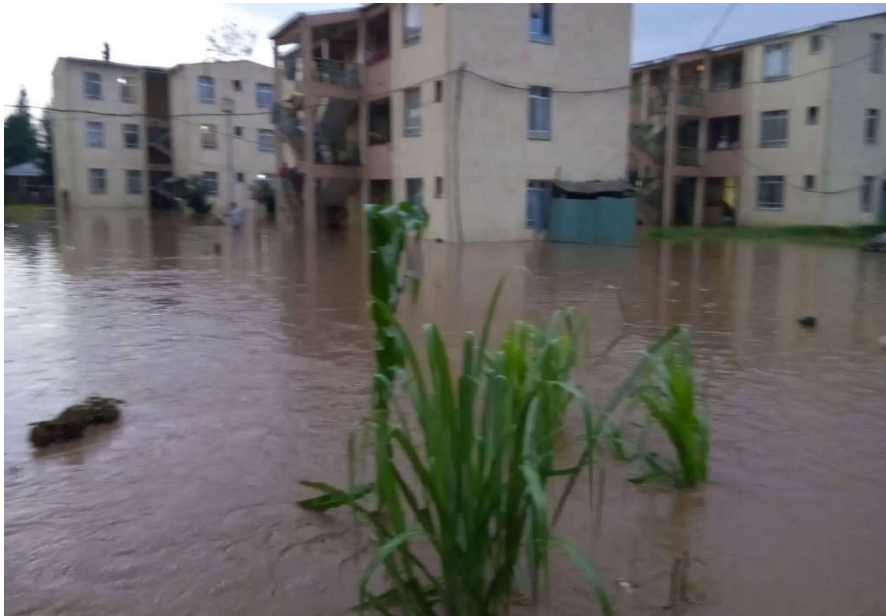
Figure 1.1: Picture Showing Flood Damage occurred May, 27, 2018 Dippo Condominium.
