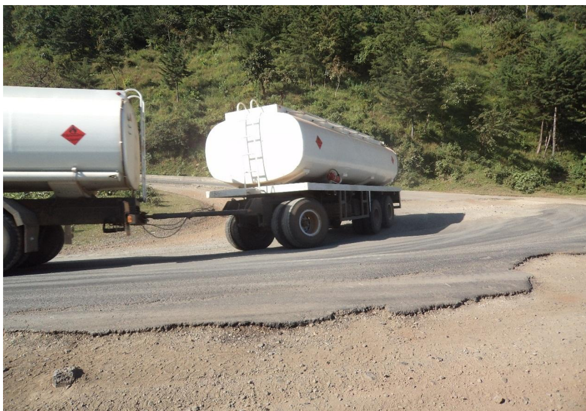
Photo: Switch-back Curve Having Radii of 13.75m in Correspondence with 5.83% grade Found in Sokoru Woreda (Shoshe) At Station Km 247+820.
