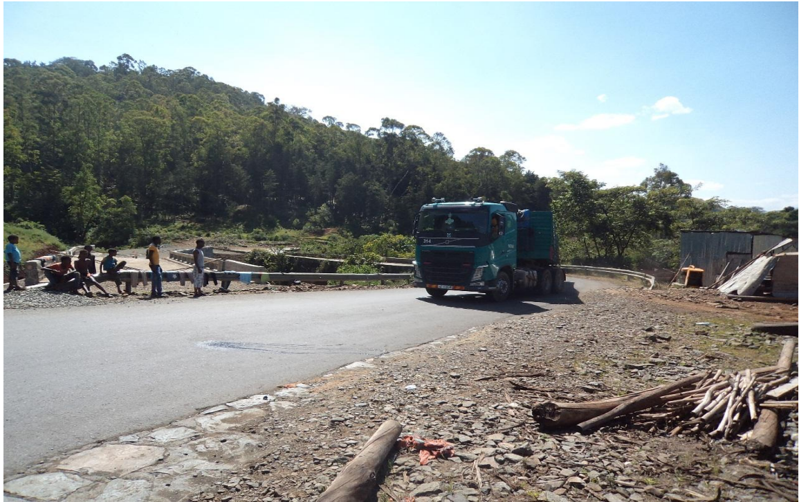
Photo: Kosho Bridge both Existing and Re-located Bridge
