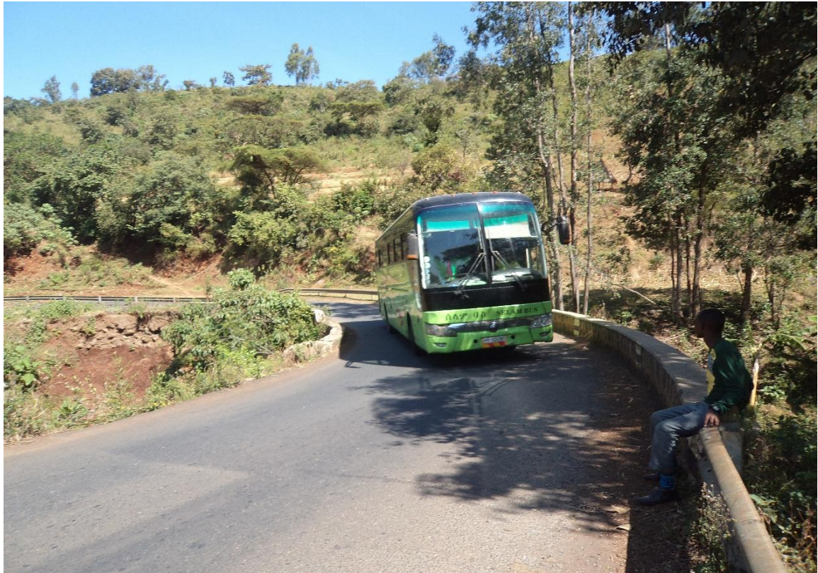
Photo: Narrow (6m) Bekere River Bridge Found in Sharp Horizontal Curve (Curve Radii 26m) in Sokoru Woreda at Station Km 247+216
