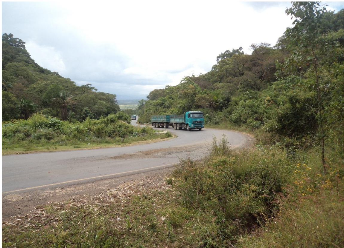
Photo: Steep Downgrade of 7.865% in Correspondence with Successive Sharp to Reverse Curves (Consisted of Radii 31m) at Beda-Buna Approach Jimma Town.
