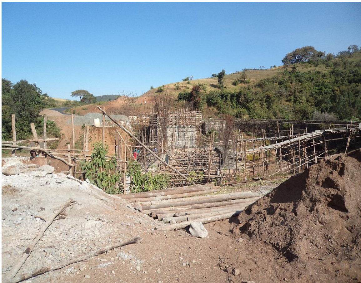
Photo: Simini Bridge both Existing and Re-located Bridge
