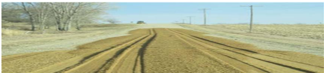
Figure 2.8 Good example of evenly dumping gravel on the road
