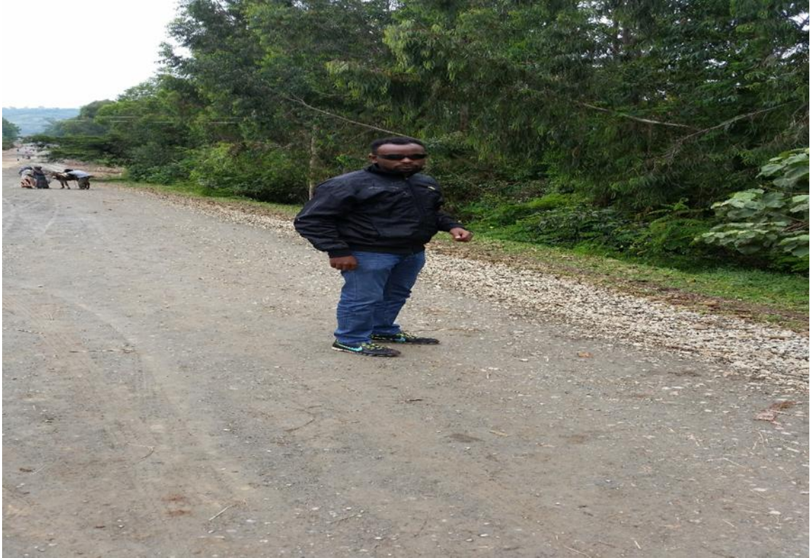
Gravel road performance observation
