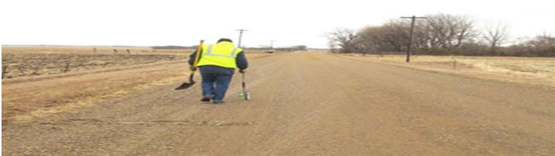
Figure 2.7 Very good practice of measuring and marking spread distance
