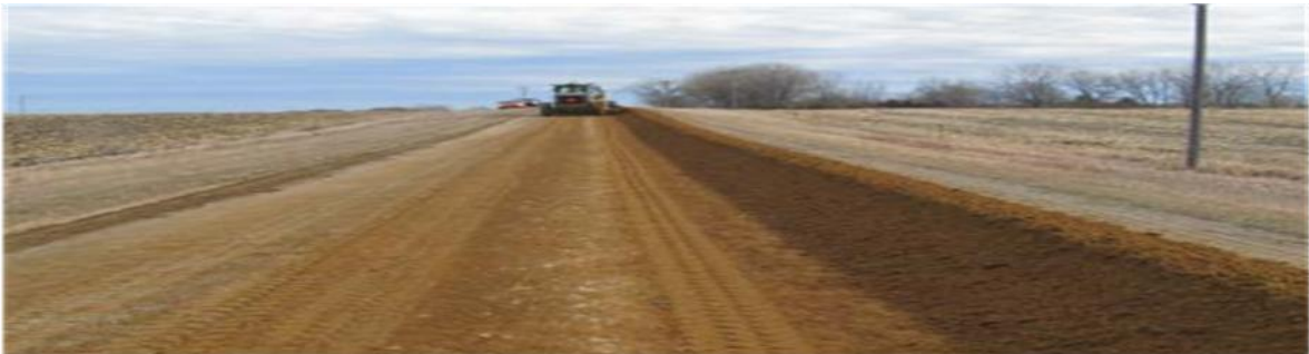
Figure 2.10 windrowing and equalizing the new gravel
