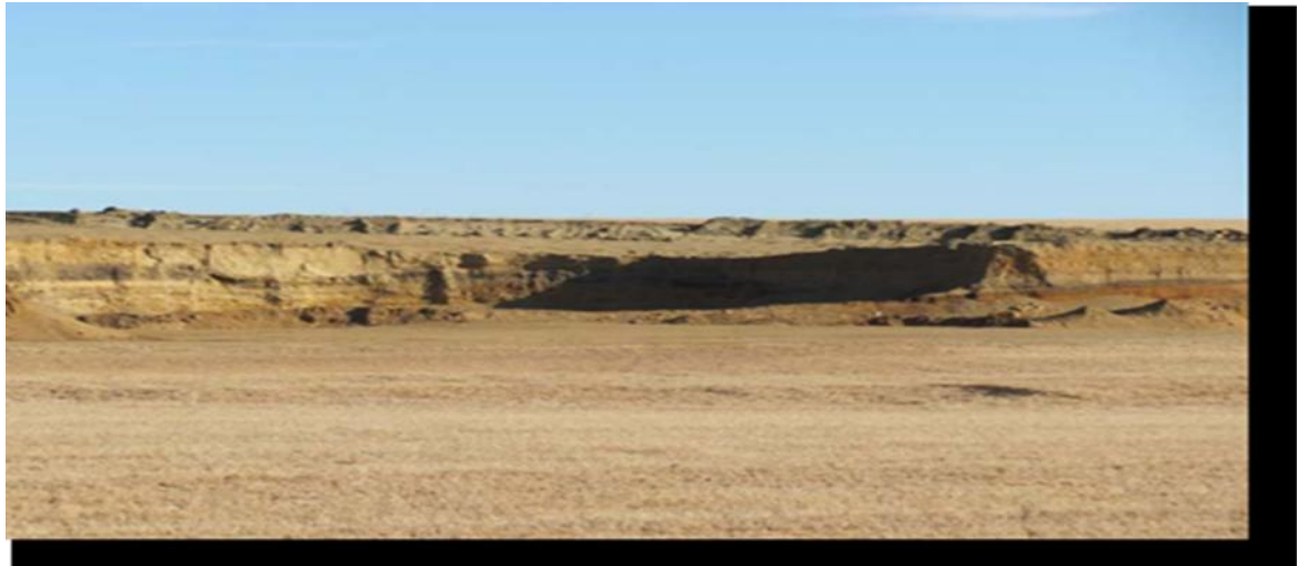
Figure 2.4 Good example of top soil and vegetation stripped
