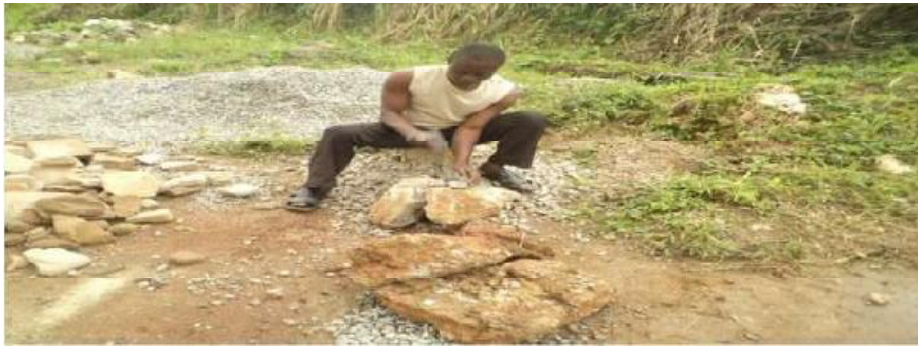
Figure2.7: Showing the process of breaking the demolished concrete [26].
