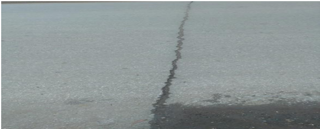
Figure 3. 9: High severity of block cracking (June, 2018)
