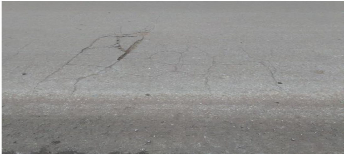
Figure 3. 7: Low severity block crack (June, 2018)
