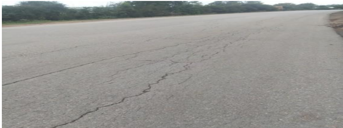
Figure 3. 7: Low severity block crack (June, 2018)
