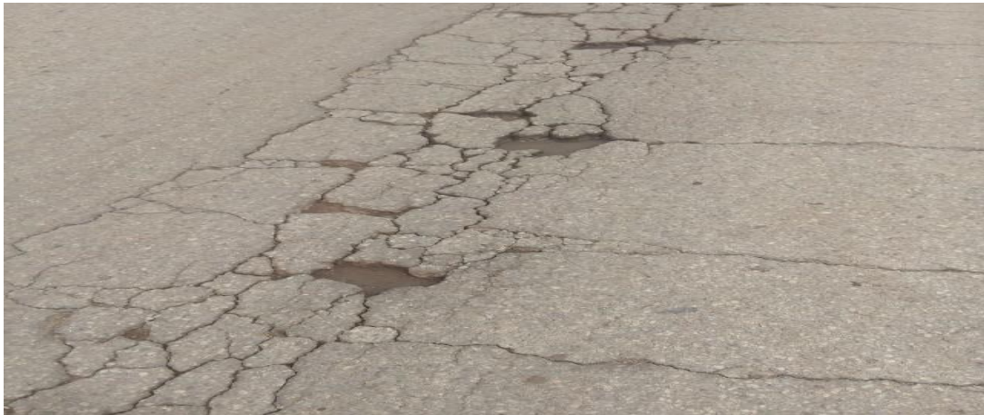
Figure 3. 9: High severity of block cracking (June, 2018)
