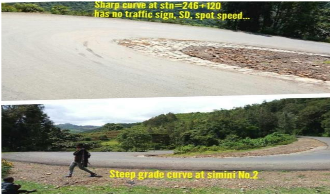
Figure 4.8: Curve with a Problem of Grade, Sharpness (Aug. 02/2011 by Dereje)
