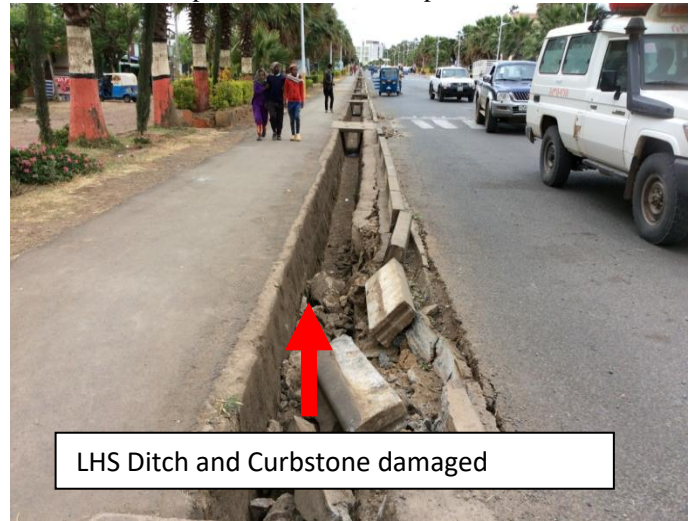
Wereba Town Concrete Ditch failure view
