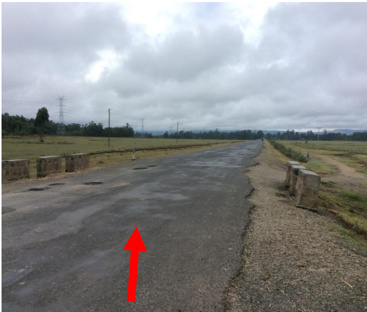
Mare Zone to Doyogena Town Potholes on Pavement @ Coordinated (37.791227E, 7.37548N, 2399m)
