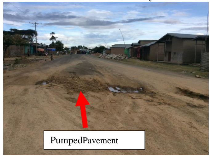
Wereba Town shoulder and RHS Masonry Ditch Failure
