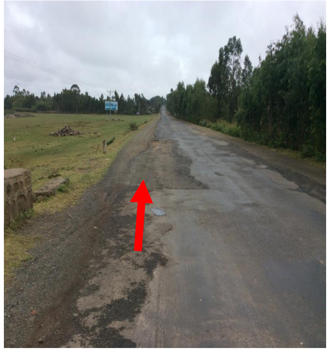
@ Hossanato Mare road Corrugated Pavement @ 0+248km Coordinated (37.821246E, 7.433378N, 2210m)
