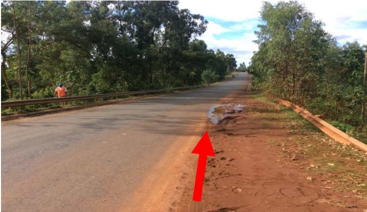
Figure 12:-Sodo Town Pavement
