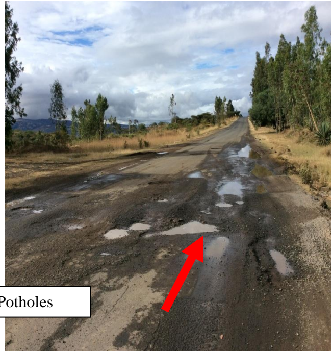
@ Alkaso Town pavement failure and pot holes
