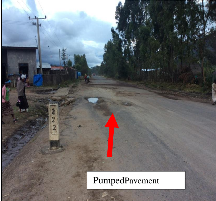
Fonka Town Pavement Carriageway Failure @ 0+222km Coordinated (37.961151E, 7.643239N)
