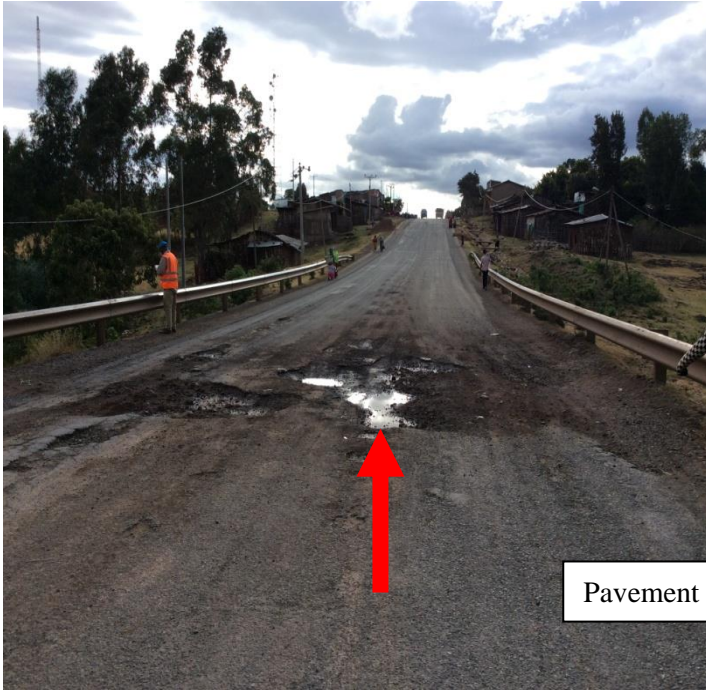
@ Silita Zone Meneharya City bridge pavement layer failure
