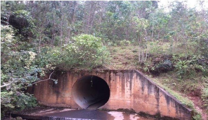
Sodo town steel pipe culvert @ 0+323km Coordinated (37.470936E, 6.879384 N, 1939m)
