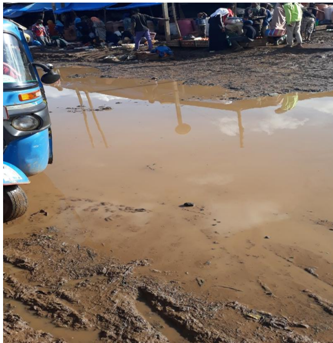
Figure 4.6 inlets closed by silt and mud ( source: field survey ).
