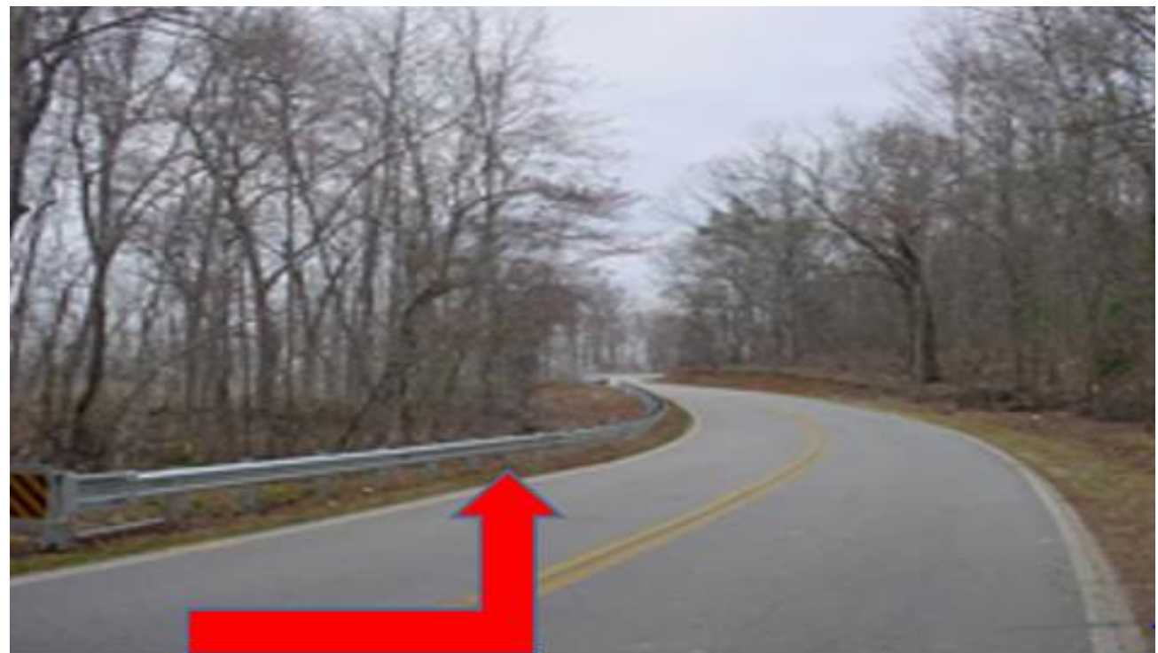
Figure 1 Guard rails and pavement materials provided at curves (source =Road safety audit hand book)
