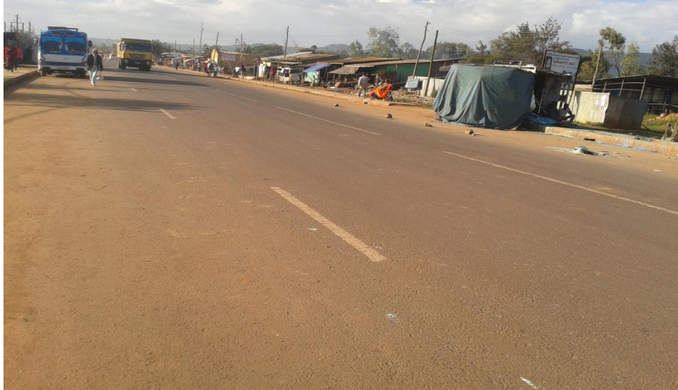
Figure 16 Property damage due to RTAs near Shenen Gibe Hospital
