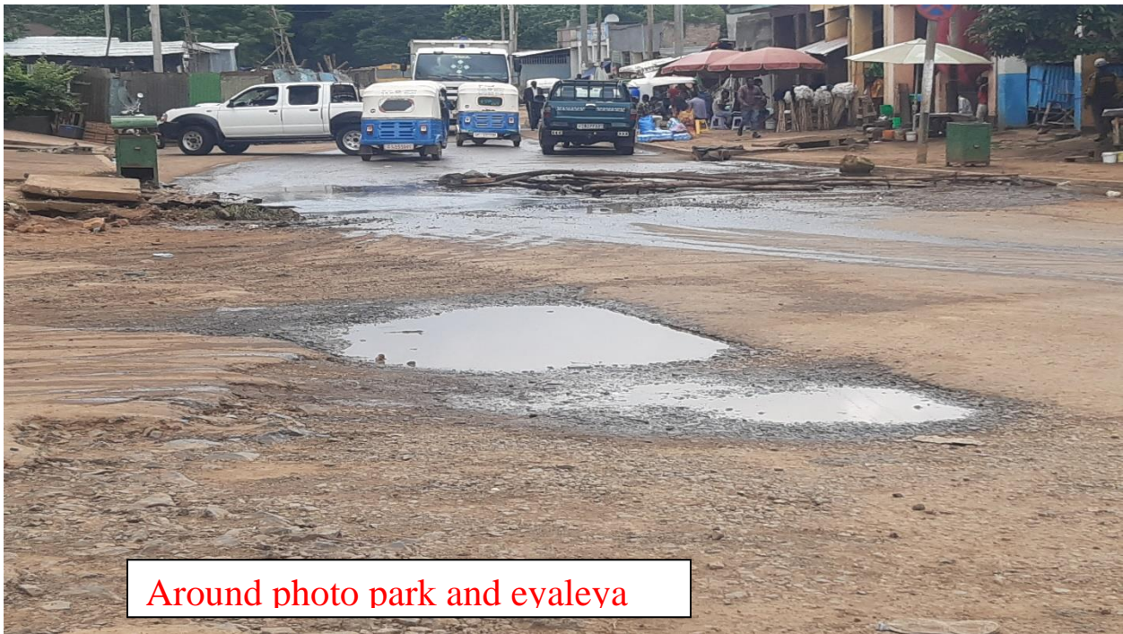
Figure 5. Absence of storm water drainage facility
