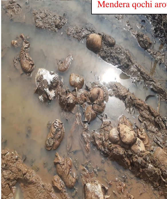
Figure 13. Stagnation of water due to absence of proper drainage
