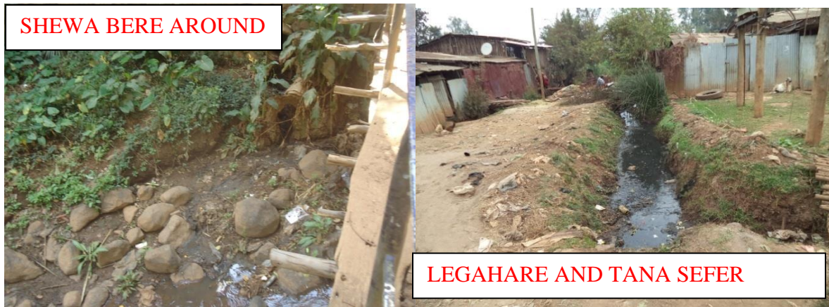
Figure 10. Liquid wastes are connected with storm water drainage lines
