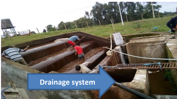
Figure 3.3: Aeration (cascade) (photo taken on 2 August, 2019)
