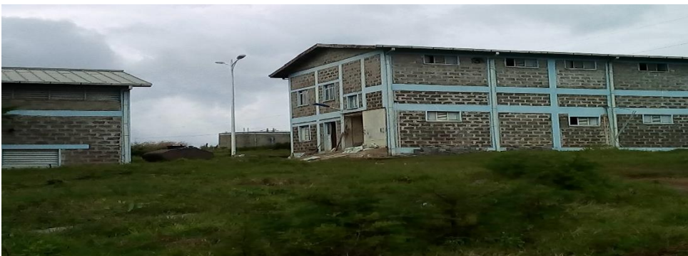
Figure N-3: Chemical building
