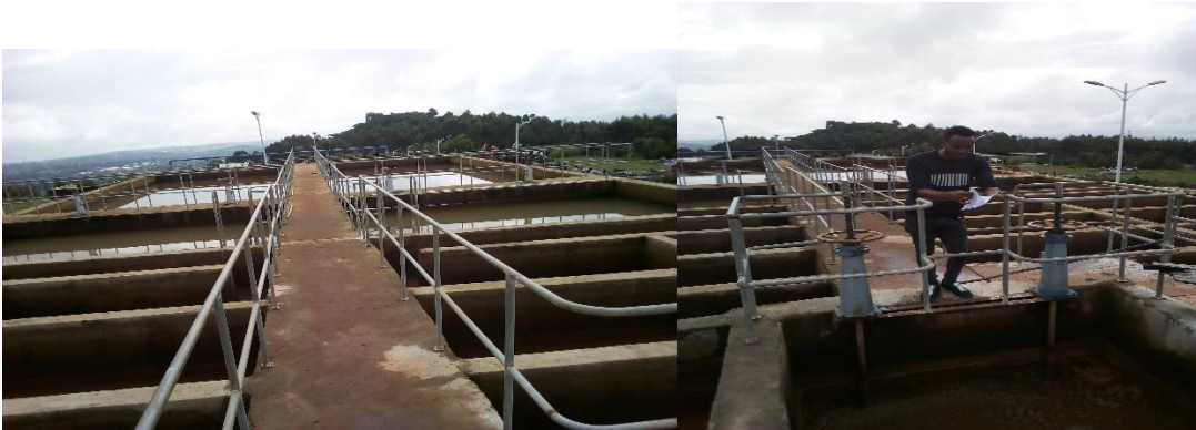
Figure N-1: WTP
