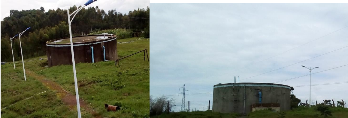
Figure 4.1: The existing service reservoirs (Source: field observation, August, 2019)
