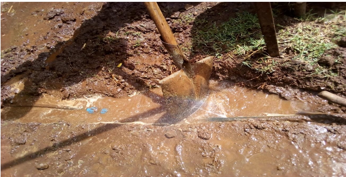
Figure 4.13: Pipe bursting (Source: field observation, August, 2019)
