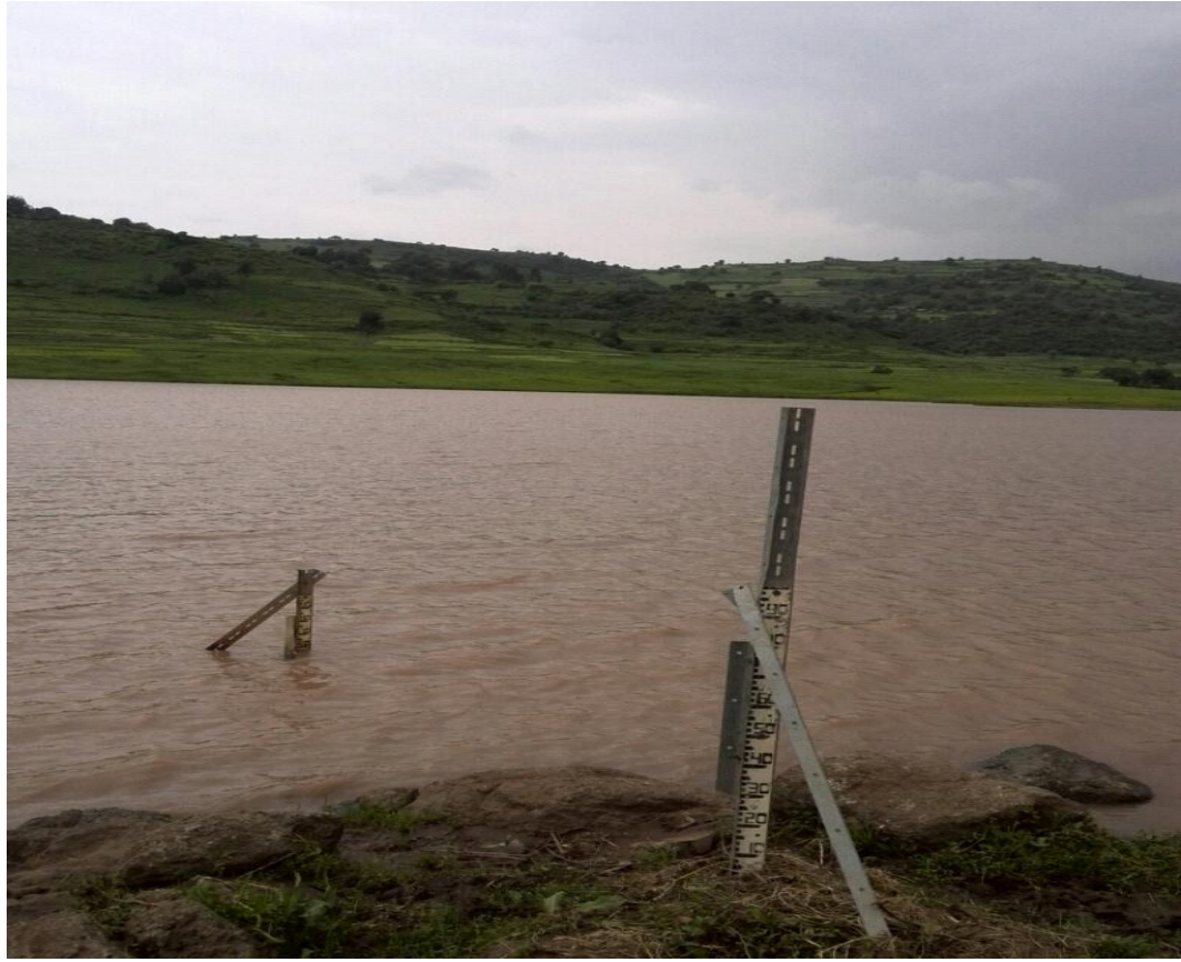
Figure3.11 Partial view of Gomit reservoir and staff gauge (source site visit)
