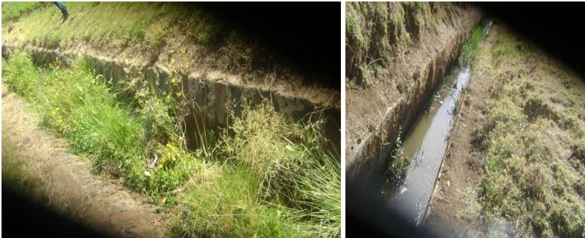
Figure4. 21 canal condition of Gomit irrigation project
