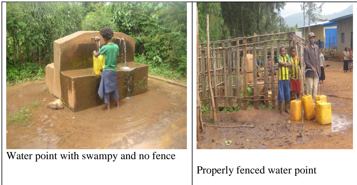
Figure4.12 Stages of water points after construction
