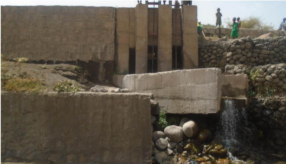
Figure 5: Gate of the weir
