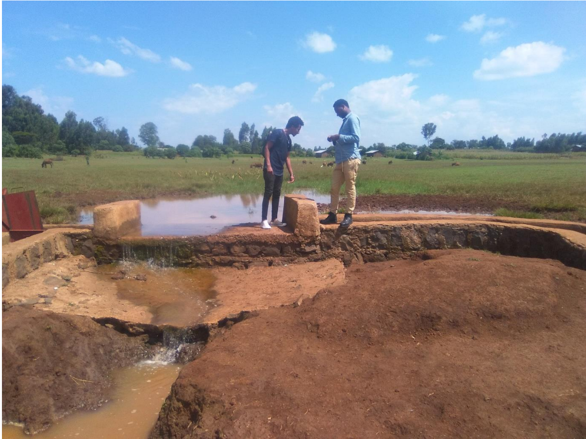
Figure 4.3 cross drainage structure
