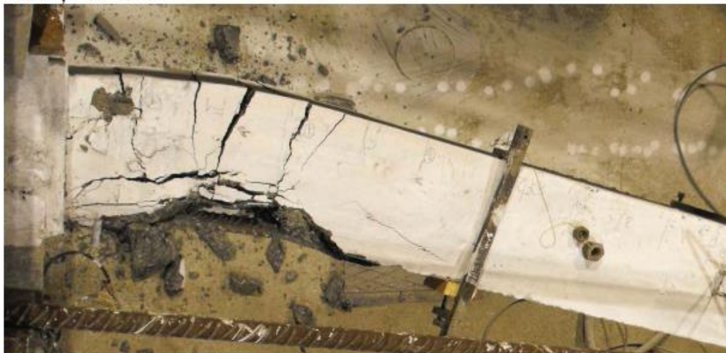
Figure 4.30: Failure mode of column under experiment (Campian et al., 2011)
