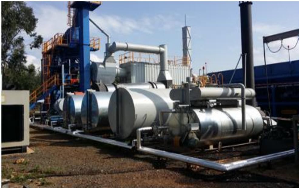
Figure 8: Asphalt storage tanks
