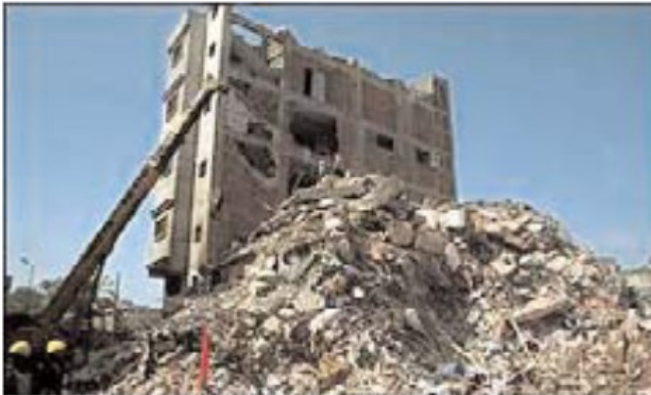
Figure 2.14: Collapsed textile factory in Alexandria, Egypt (BBC News, 2000)
