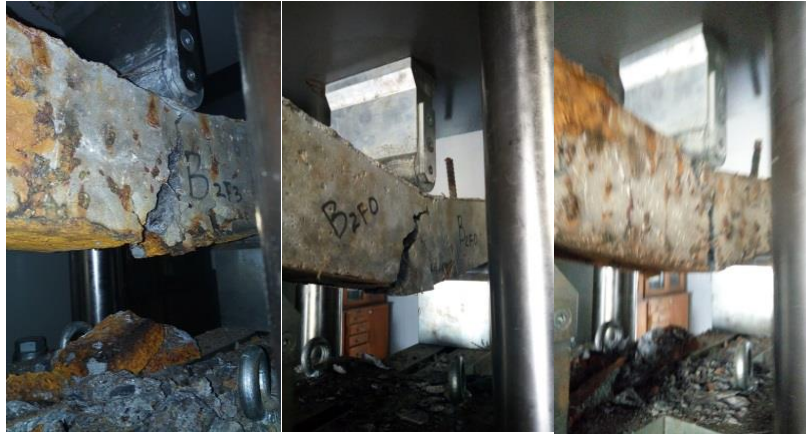
Figure 4. 23: Corroded SFRC beam failures.
