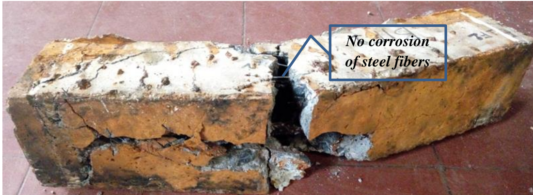
Figure 4. 19: Corroded SFRC beam after flexural strength test.
