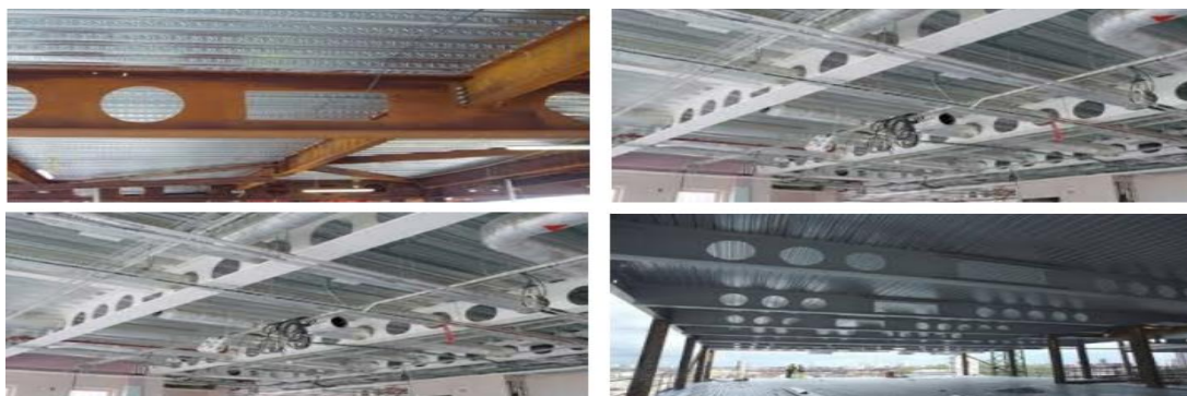
Figure 2. 1: Web openings steel beam applications [8].
