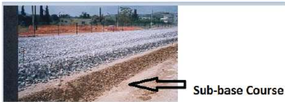
Figure 2. 6: Sub Base course layer (Umesh, 2019)
